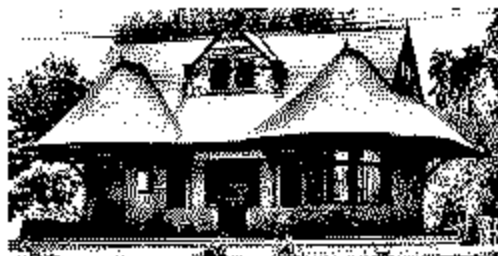
North Edgewater station (at Granville)
